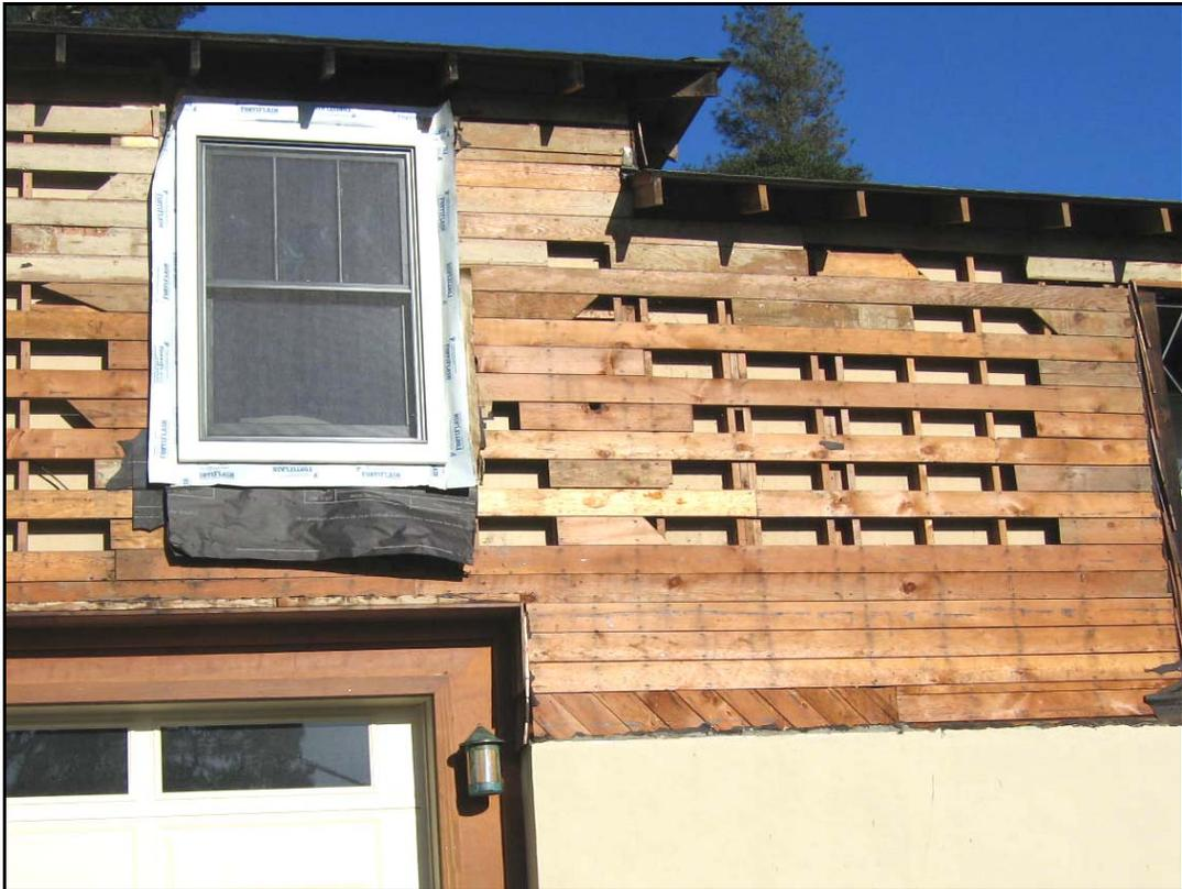
**Photo 2 – However, Removal of the Deteriorated Redwood Shakes Reveals No Water Damage at the Wood Board Sheathing or Stud Framing**
