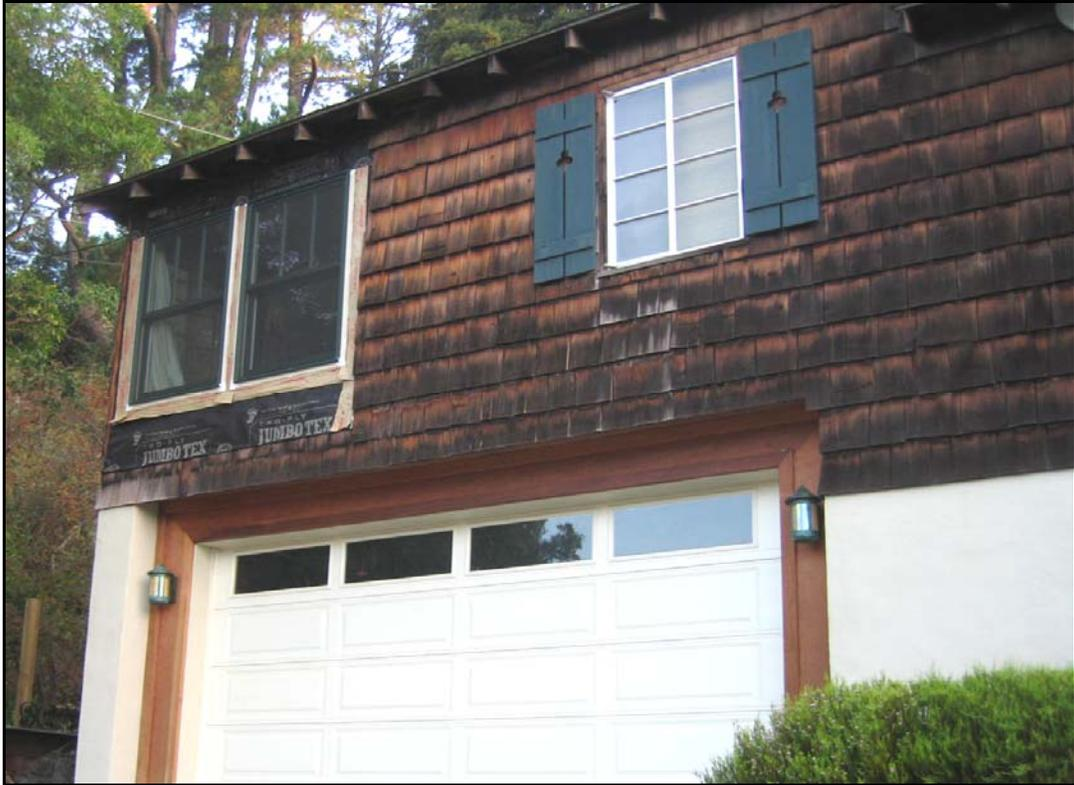
**Photo 1 – Owner Is Replacing the Original Aluminum Windows (at Right) with New Metal-Clad Wood Windows (at Left). Note the Severely Deteriorated Redwood Shakes**
