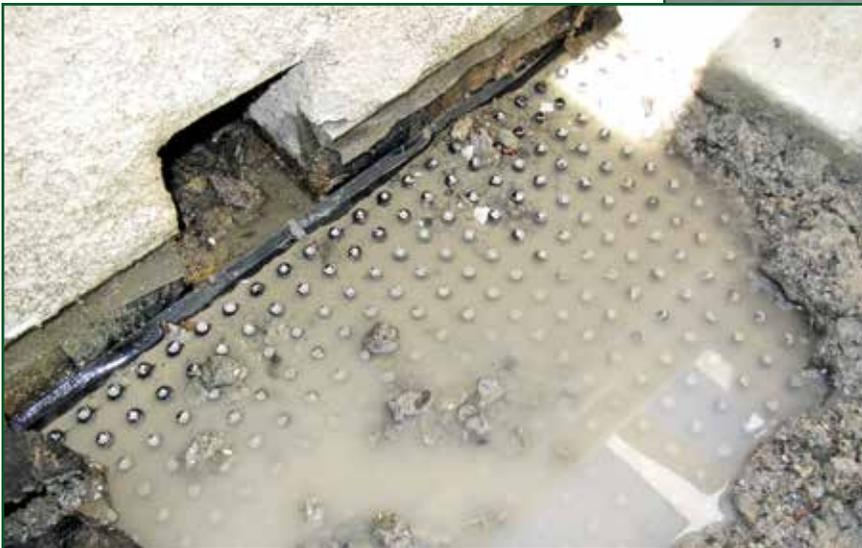
*Photo 4 – Water ponds under the deck’s concrete covering.*
