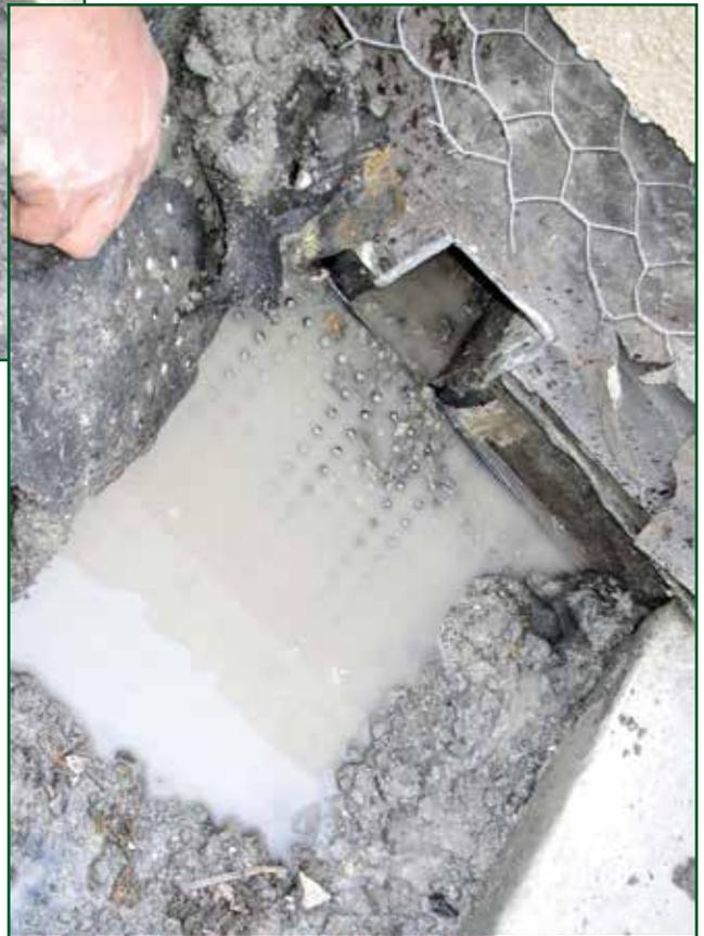
*Photo 7 – Water ponds due to negative slope and other construction deficiencies.*
