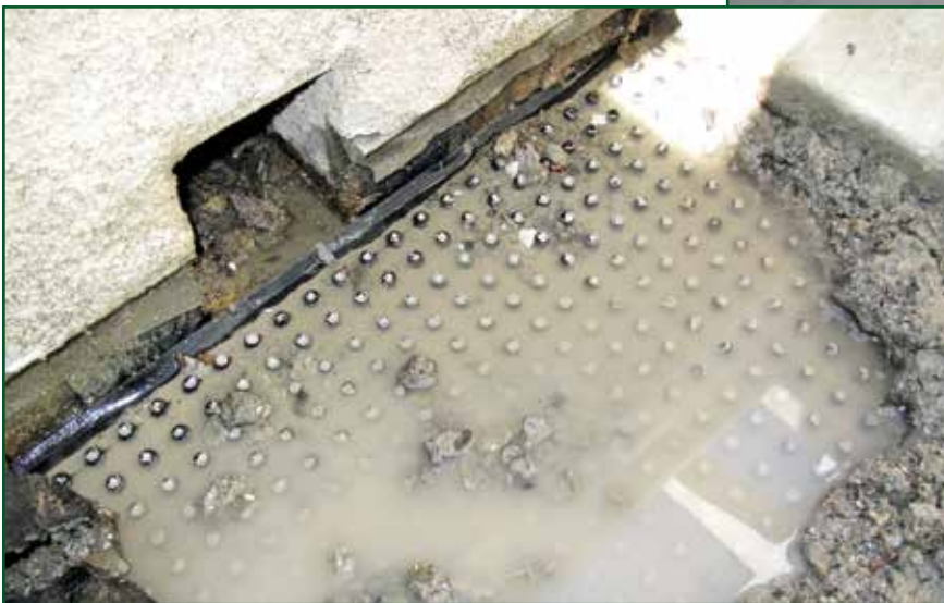
Photo 5 – Waterproofing is negatively sloped away from the scupper.
