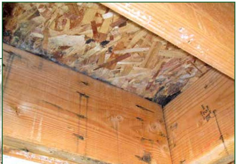
*Photo 9 – Soffit removal below another deck reveals evidence of water seepage from above.*
