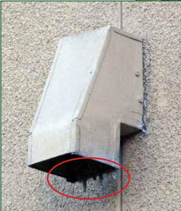
water (Photo 6) that cannot fully drain due to negative slope in front of the scupper (Photo 7), which is exacerbated by concrete debris within the scupper’s throat (Photo 8).
