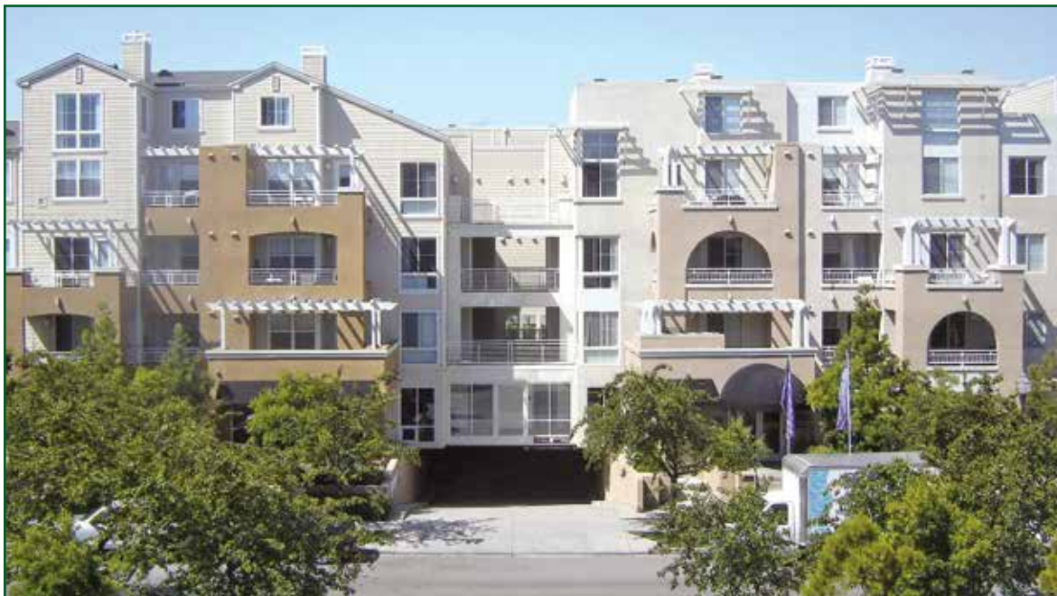
Photo 1 – The apartment complex has 187 wood-framed decks.
