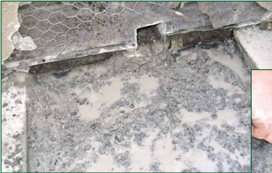
Photo 6 – Concrete removal releases a flood of trapped water.
