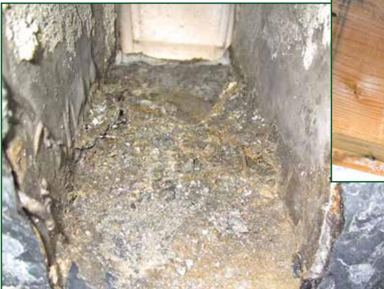
*Photo 8 – Concrete debris within the scupper's throat impedes positive drainage.*
