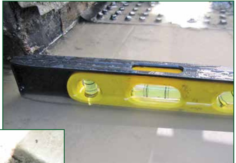
Photo 5 – Waterproofing is negatively sloped away from the scupper.
