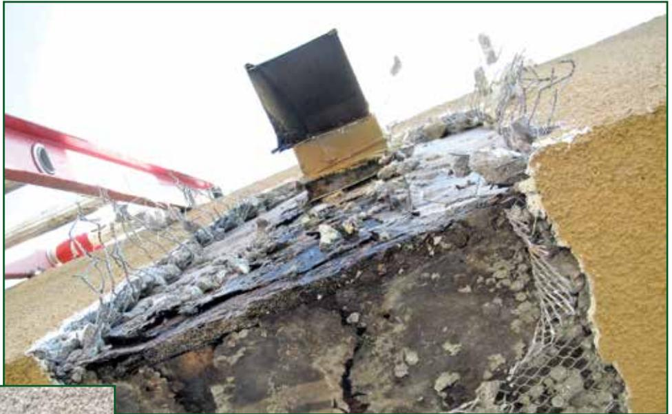
*Photo 2 – “Concrete stalactites” are evidence of slow seepage of ponded water.*
