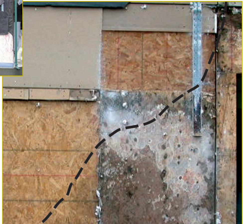
Photo 2 - Hardwood OSB sheathing with severe white-rot decay is surrounded by relatively undamaged hardwood OSB. The dashed line traces the upper limit of the migrating water. Note that the white-rot deterioration has spread upward from the water line. (The localized brown-rot decay at the upper right is spreading from underlying infestation of a softwood-framing member.)
