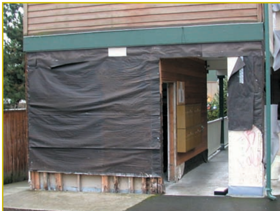
Photo 1 - Overview of the work area.
